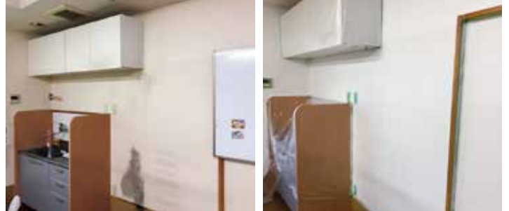
③既存壁塗装前
